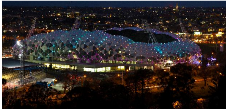
Victoria's cutting-edge AAMI Park is identified by its unique bioframe design with geodesic dome roof.
